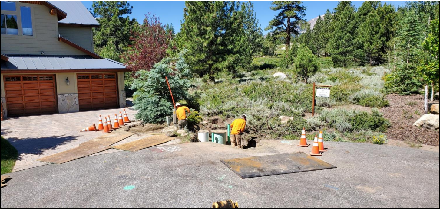
Construction crew working in meter pit in The Trails neighborhood.
