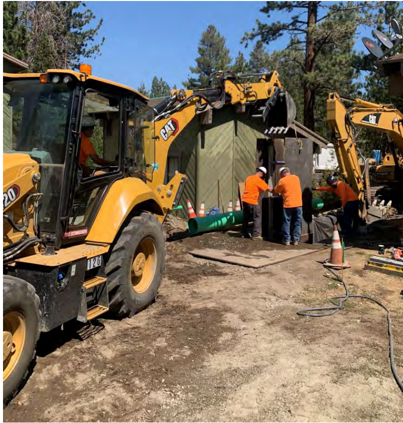
Figure 1- Crew setting up trench shoring in preparation for pipe installation
