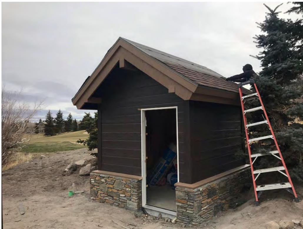
Figure 6- Building near completion
