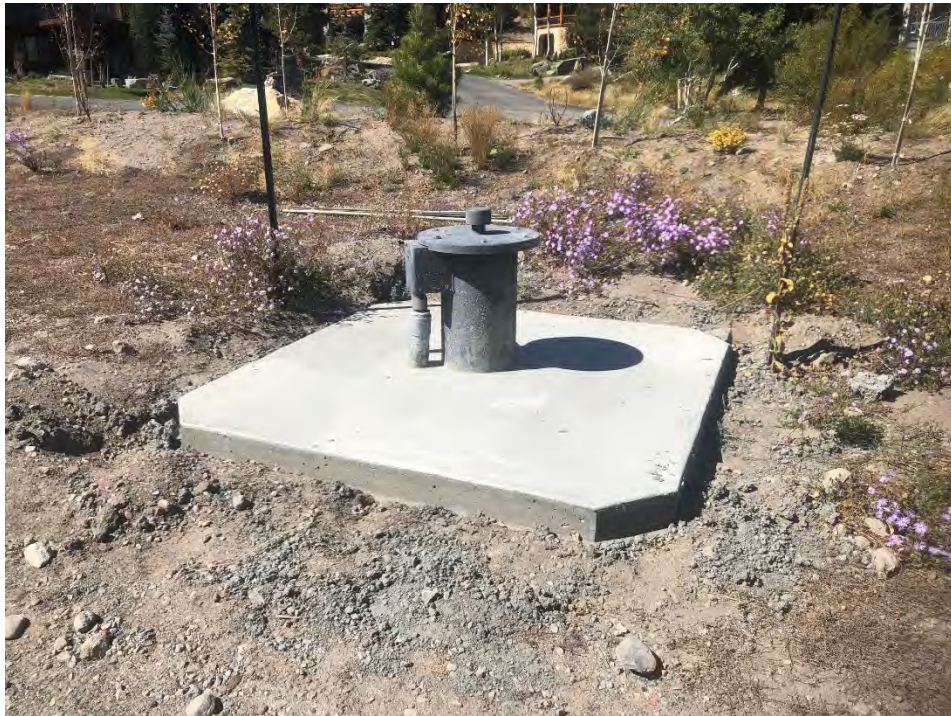
Figure 8- Well head after pouring concrete pad
