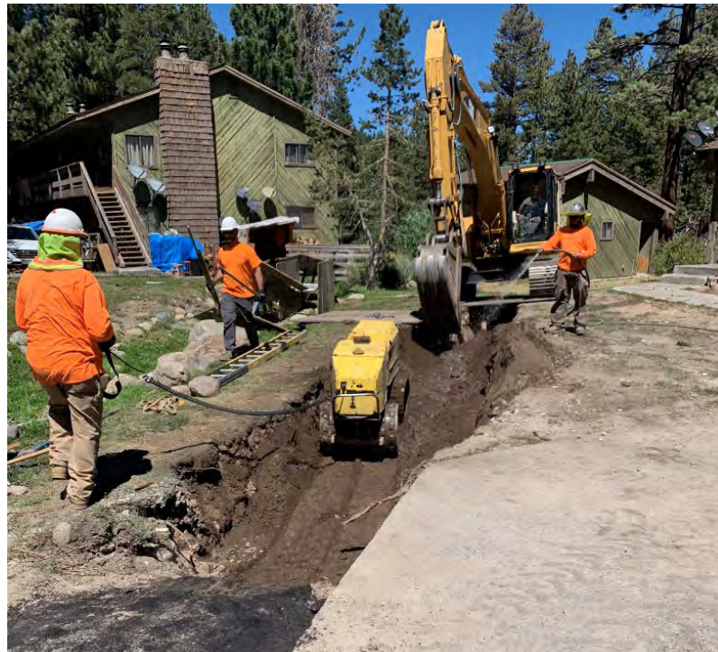
Figure 2- Crews backfilling and compacting the trench
