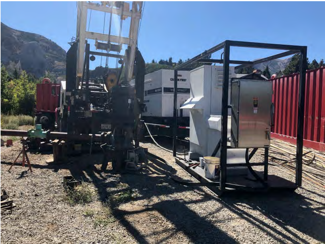
Figure 4- Carson Pump performing well development
