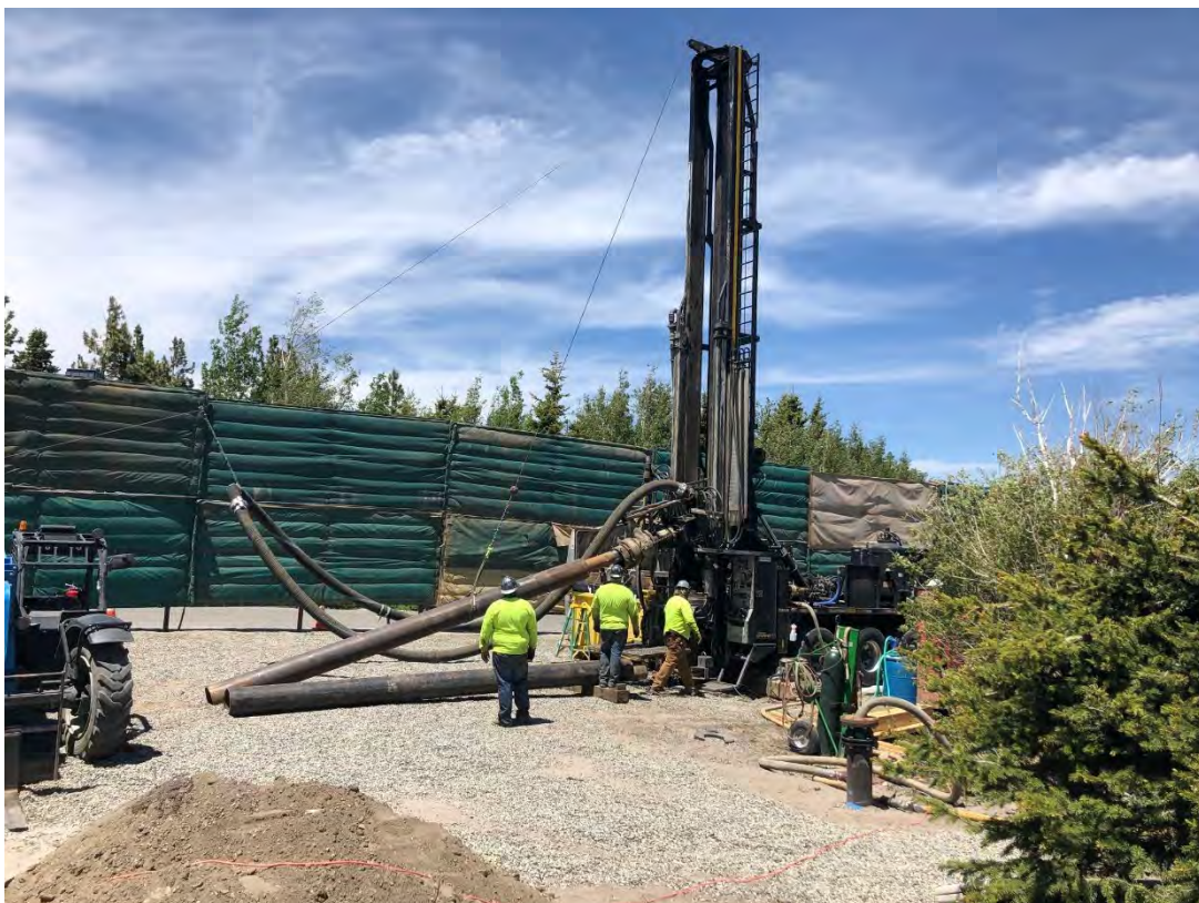
Figure 2- Adding stick of pipe to drill rig
