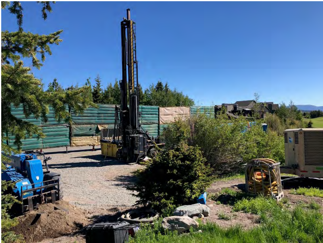
Figure 1- Well site with drill rig
