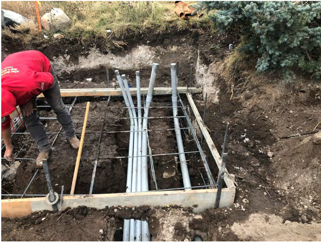
Figure 5- Allied General Contractors installing conduits for building
