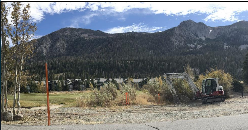
Contractor installing receiver holes for sound attenuation panels.
