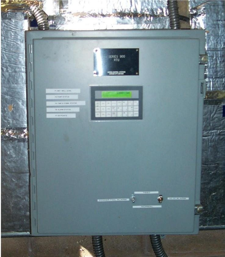
Figure 2: SCADA communication system in East Mary Lift Station
