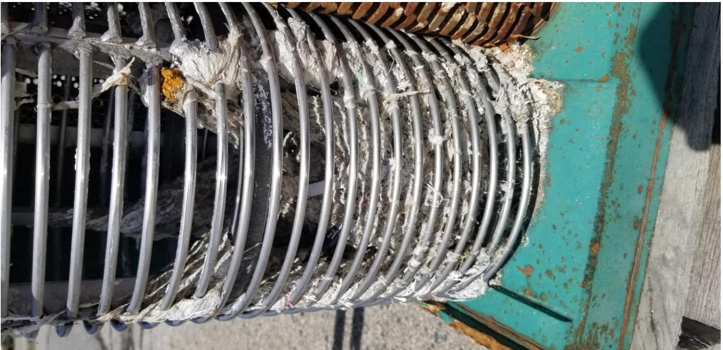
*This is a picture of the influent grinder completely clogged with wipes. The District spent over \$200,000 to replace the grinder with a trash removal system due to the persistent problems caused by the influx of wipes at the wastewater treatment plant.*
